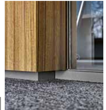
4. Junction of glass at Bridge structure showing the recessed detail
