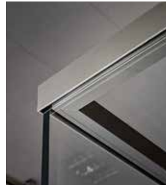
3. Top junction between glass and upper rail (incorporating cable conduit)
